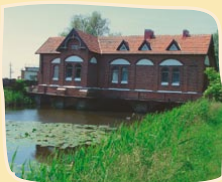
Water lifting station – the Šilutė Museum of Polders.
